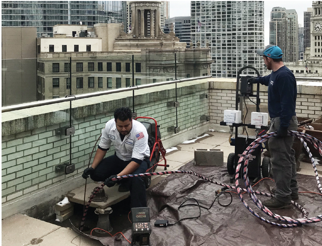
▲ American Trenchless Technologies technicians Omar Franco (left) and Andy Smith use a Quick-Coating System made by Pipe Lining Supply to fix leaks in a system of pipes—both main drainlines and branch connections—fed by roof drains atop the Old Republic Building in downtown Chicago.
